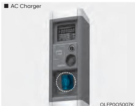
6. Connect the charging plug to the electric outlet at a AC charging station to start charging.
